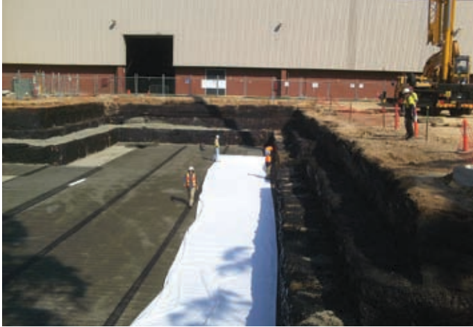
Day 1 4.00pm Grid and fabric in place.
