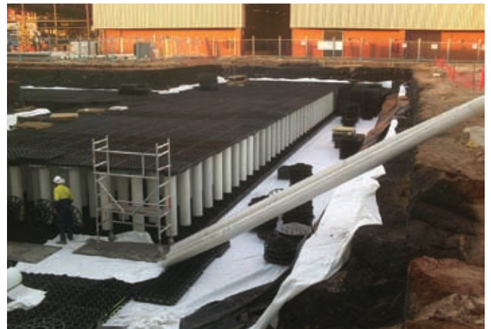
Day 5 10.15am The near completed support matrix.
