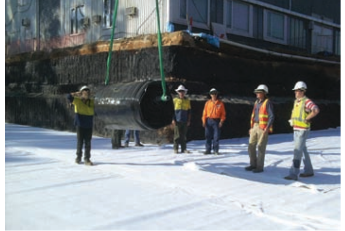
Day 1 5.30pm First liner is then rolled out.
